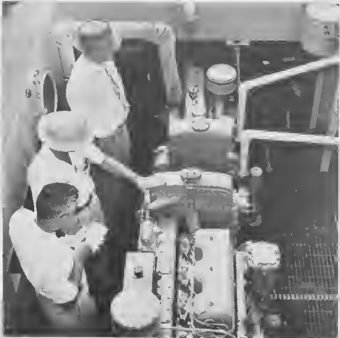
EASY ACCESS to the boat's engines simplifies repairs. Howard Garig, Marine Department, center, explains the system to Bill Hochstuhel, Public Relations, left, and Captain Larson, port captain for Esso Shipping.
